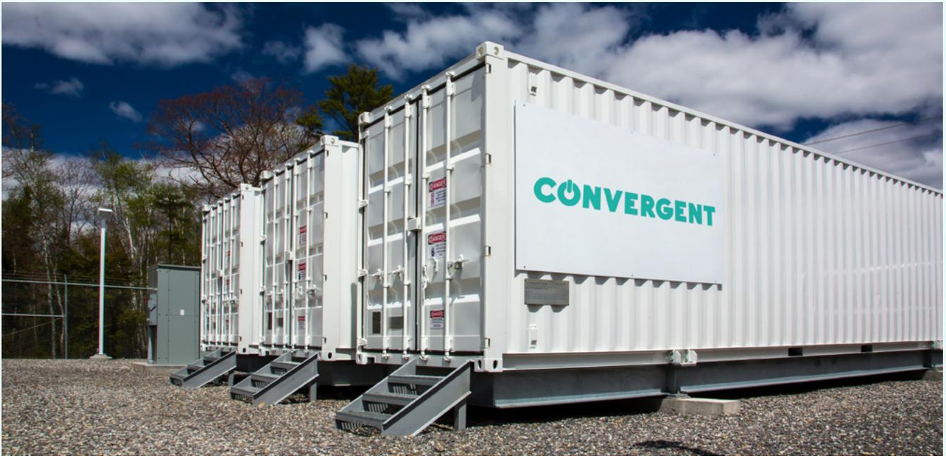
Convergent's NWA energy storage asset in Boothbay, Maine was utilized by Central Maine Power for three consecutive summers, providing on-demand power during summer peaks and preventing further deterioration to the constrained upstream transmission feeders and substations.
